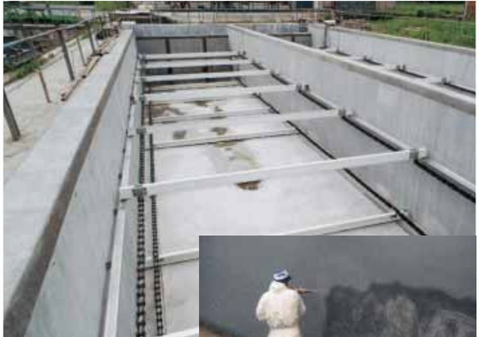
Spray application VANDEX POLYZEM Z
