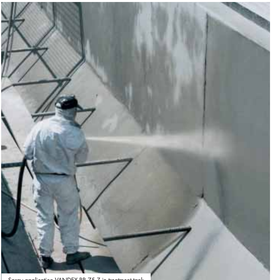
Spray application VANDEX BB 75 Z in treatment tank
