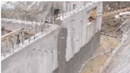
VANDEX CEMELAST as external waterproofing.
