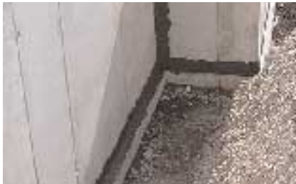
VANDEX CONSTRUCTION JOINT TAPE external application at horizontal and vertical construction joints.
