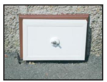
'When I get a message from the Agency's AVM flood warning service I simply fix a frame around each airbrick and then screw on the cover - it only takes a few minutes'.
